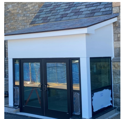
Vestibule Entrance in the main Parking Lot.
