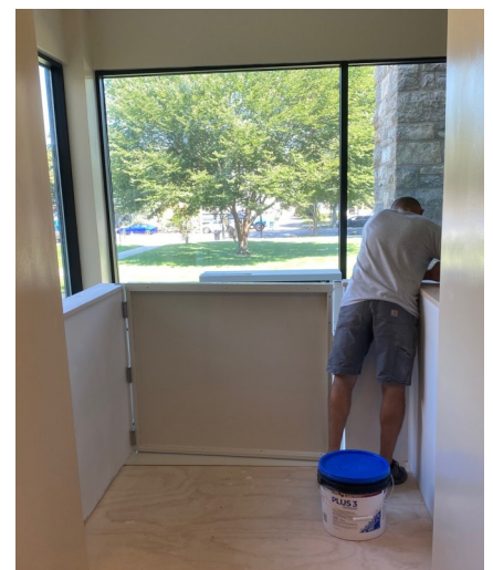
To the right upper photograph is the new lift under construction seen from the chapel narthex.
