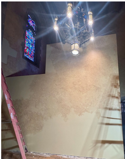
Faux painting of new elevator sheetrock walls to match the paint on existing sanctuary walls.
