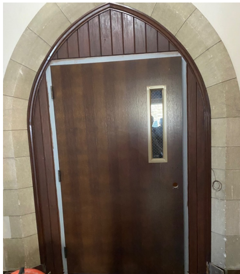
New millwork installed surrounding a new fire rated door into sanctuary from the chapel narthex. The gray metal frames and window frame will be painted to match.
